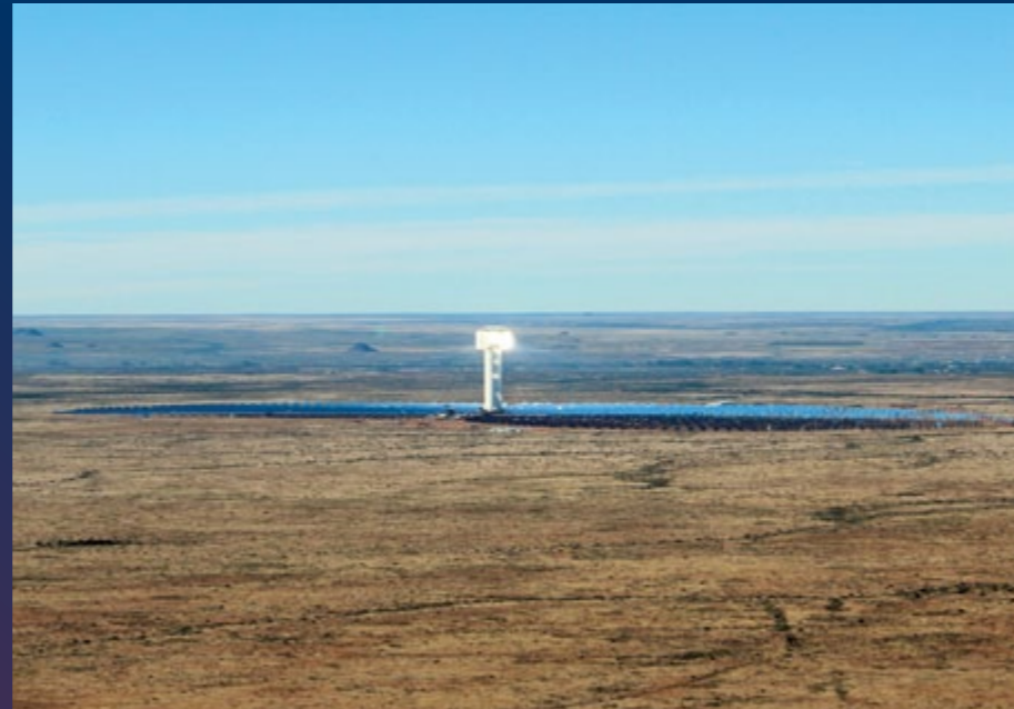
Solar Farm near Upington
